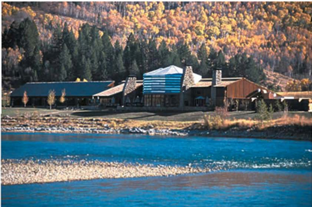
One of the major efforts at the site was to stabilize the river banks, which had been badly eroded during a flood. Tall trees shield the lodge from a nearby roadway.
