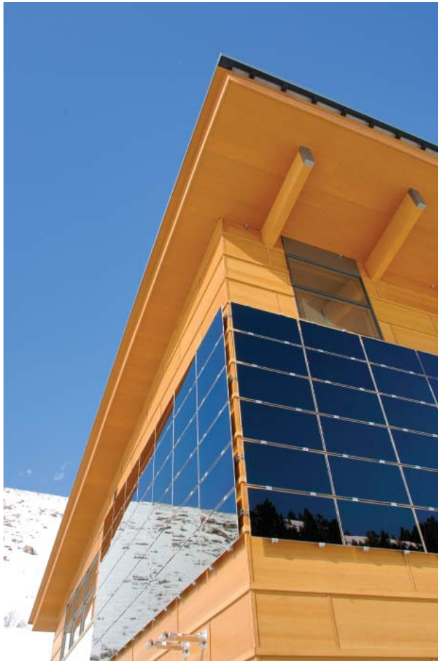
Fiber cement siding is contrasted by a vertical photovoltaic curtain wall. This is in keeping with the aspirations to both maintain traditional rural character and emulate the West's historic adaptation of technological innovation. © Mithun
